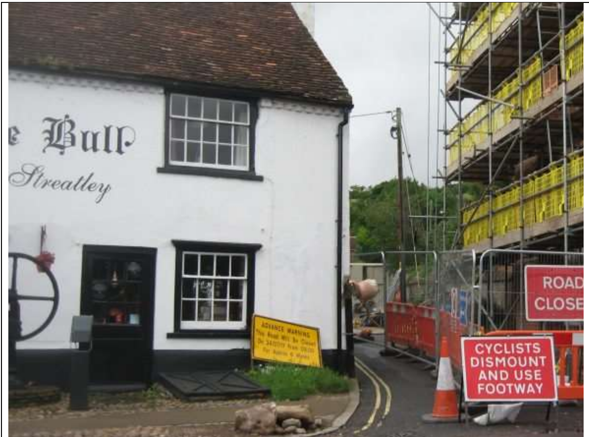
Approach from the B4009. Road closed due to repairs needed after HGV collided with Listed property and became wedged in the road.
